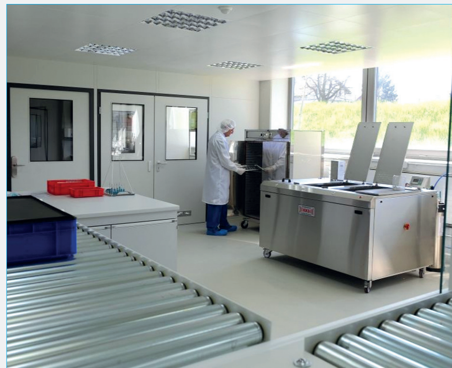
Parts cleaning in separate section
