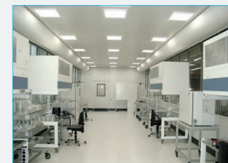
Clean room ISO 8 with flow boxes
