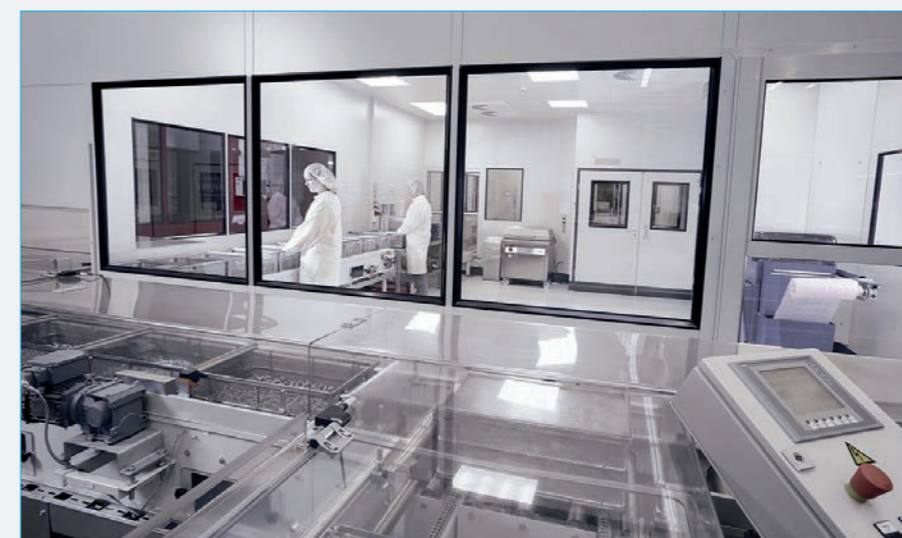
Encapsulated conveyor belts with connection to clean room
